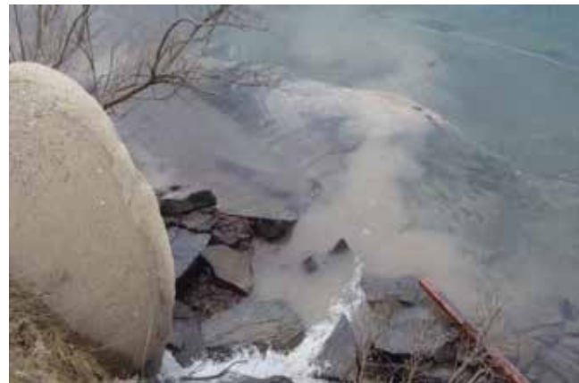
Of the 39 Rte. 219 culverts, FoDCL found 19 which directly dump run off into the lake. At this culvert outflow you can see winter road treatment and chemicals are flowing into the lake.
